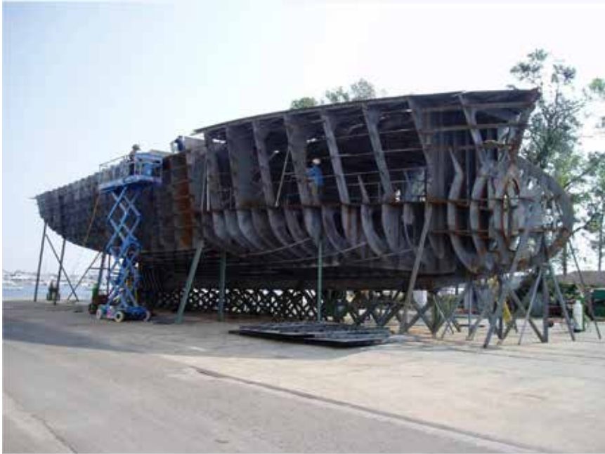
Freezer Longliner steel boat "Bering Leader" under construction at Patti Shipyards in Pensacola
